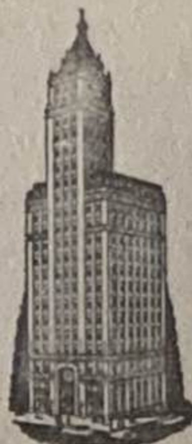
Home Office Building
